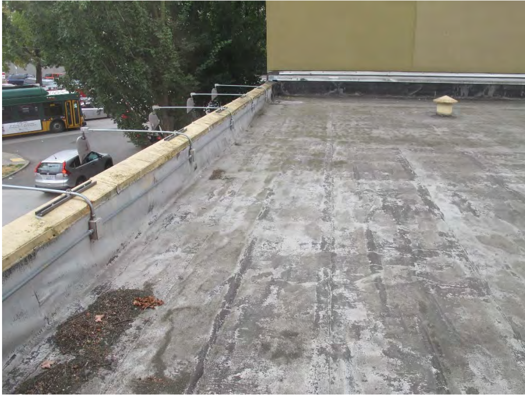
Fig. 67 – Roof of first floor portion.
