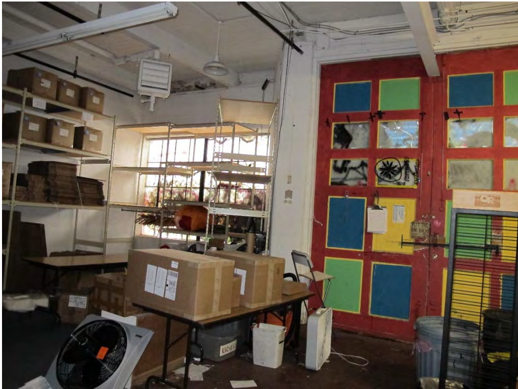
Fig. 90 – Interior, storage space in southwest building corner.
