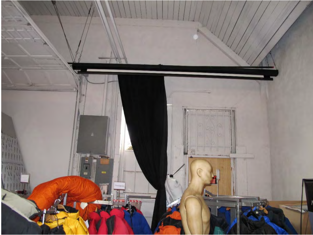
Fig. 87 – Interior, storage space in northwest building corner.
