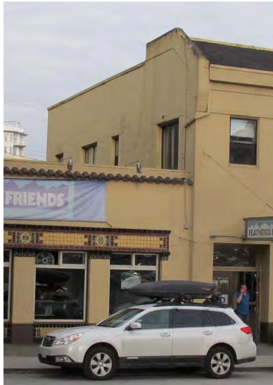
Fig. 57 – South elevation of second floor, partial view.
