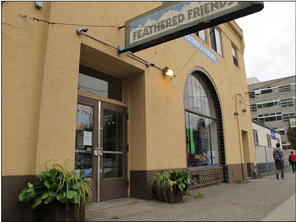
Fig. 45 – East elevation, detail
