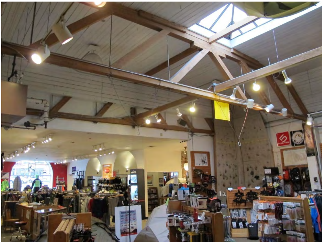
Fig. 82 – Interior, retail space in north central part of building.
