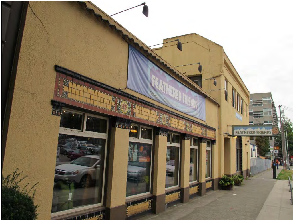
Fig. 51 – East elevation, detail of tile.
