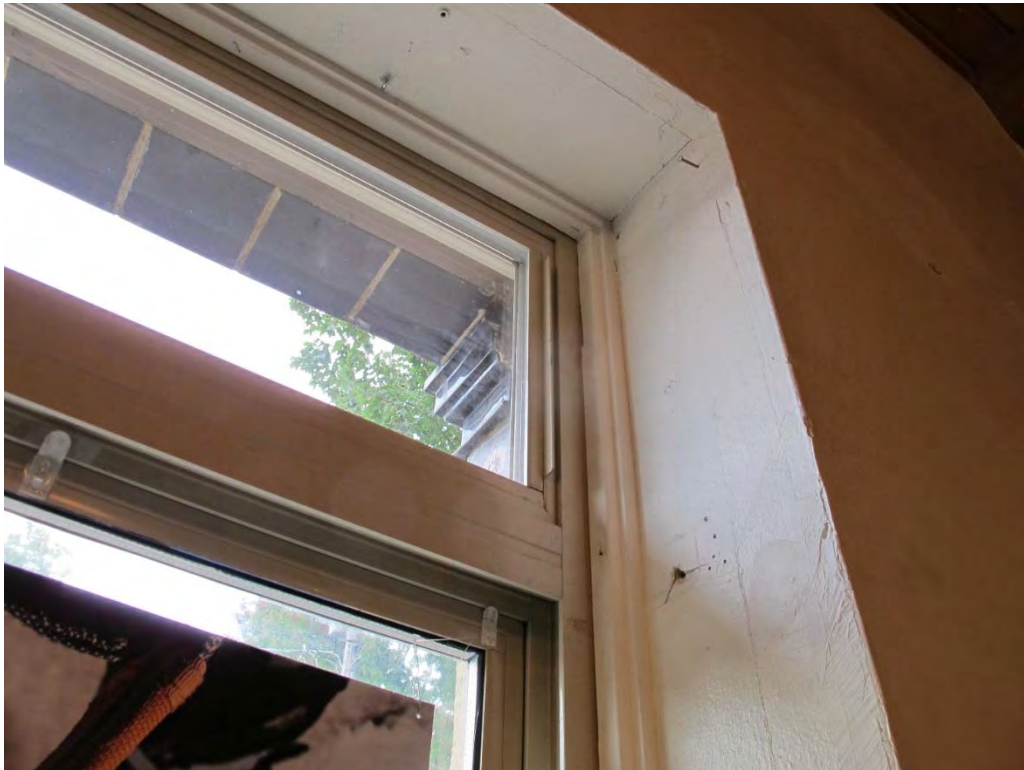
Fig. 74 – Interior, retail space in southeast building corner, detail of window.
