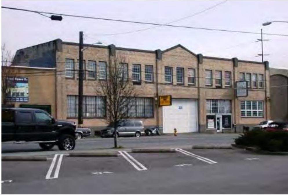
Fig. 33 – American Radiator & Standard Sanitary Corporation (1931) at 1534 First Avenue South. (DON photo)
