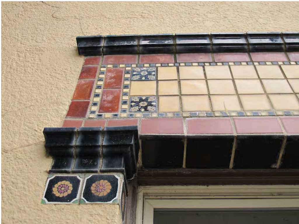
Fig. 56 – East elevation, detail of tile.
