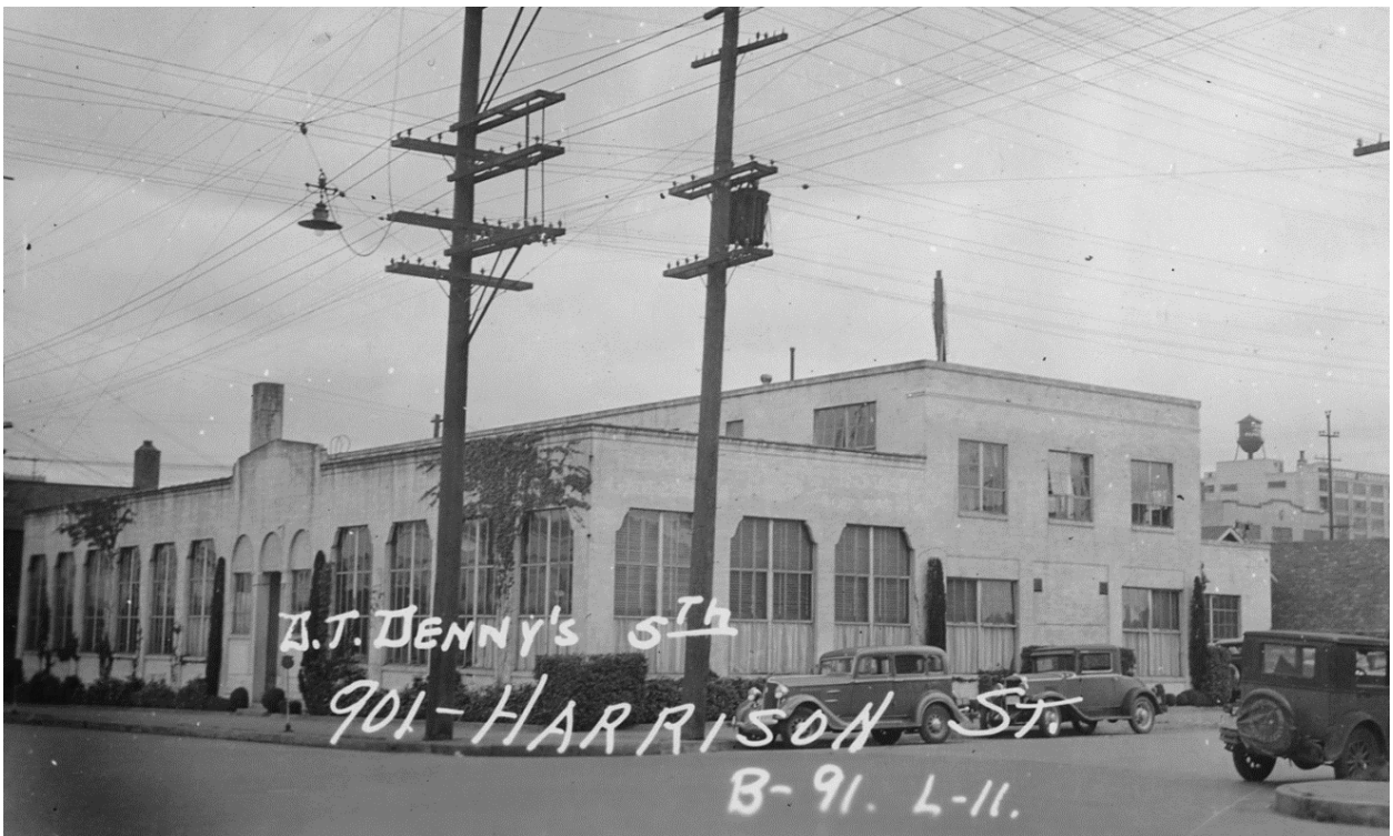
Fig. 32 – Pioneer Sand & Gravel (1927) at 901 Harrison Street, a designated Seattle landmark. (King County Tax Assessor)
