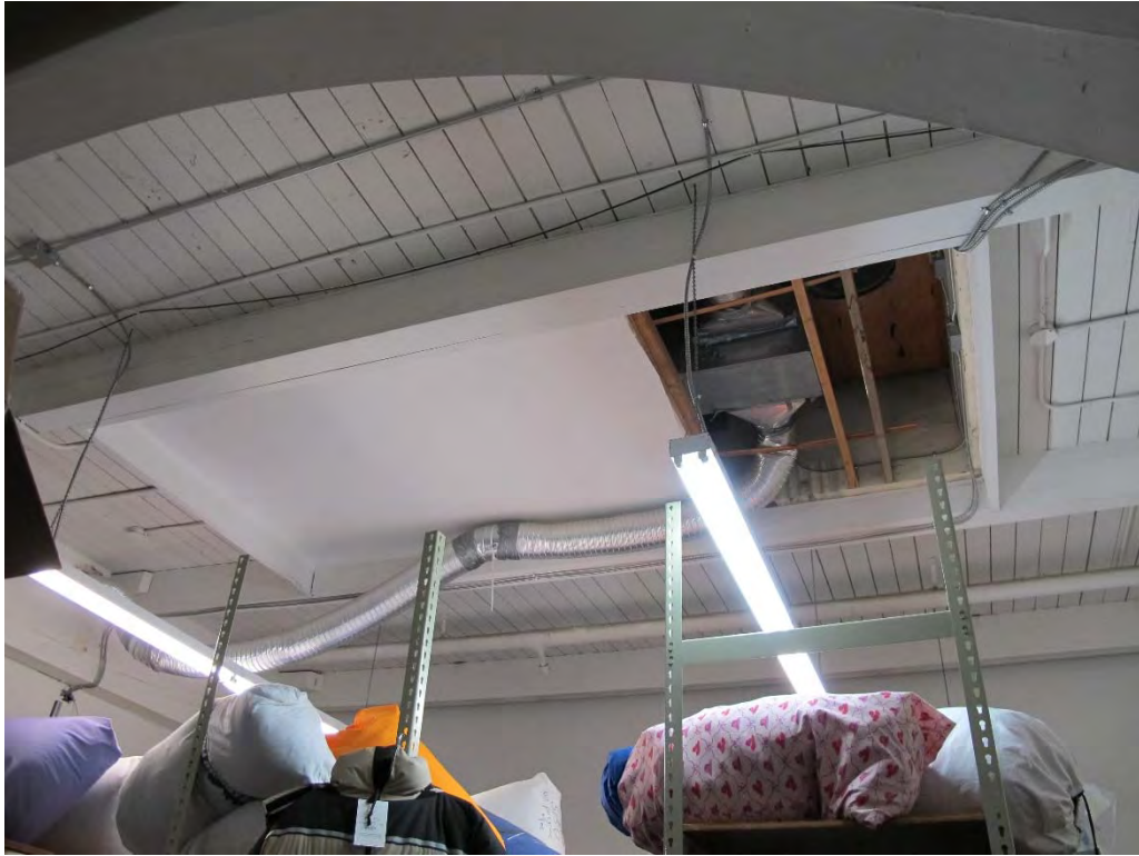
Fig. 89 – Interior, storage space in south central part of building, showing former skylight.
