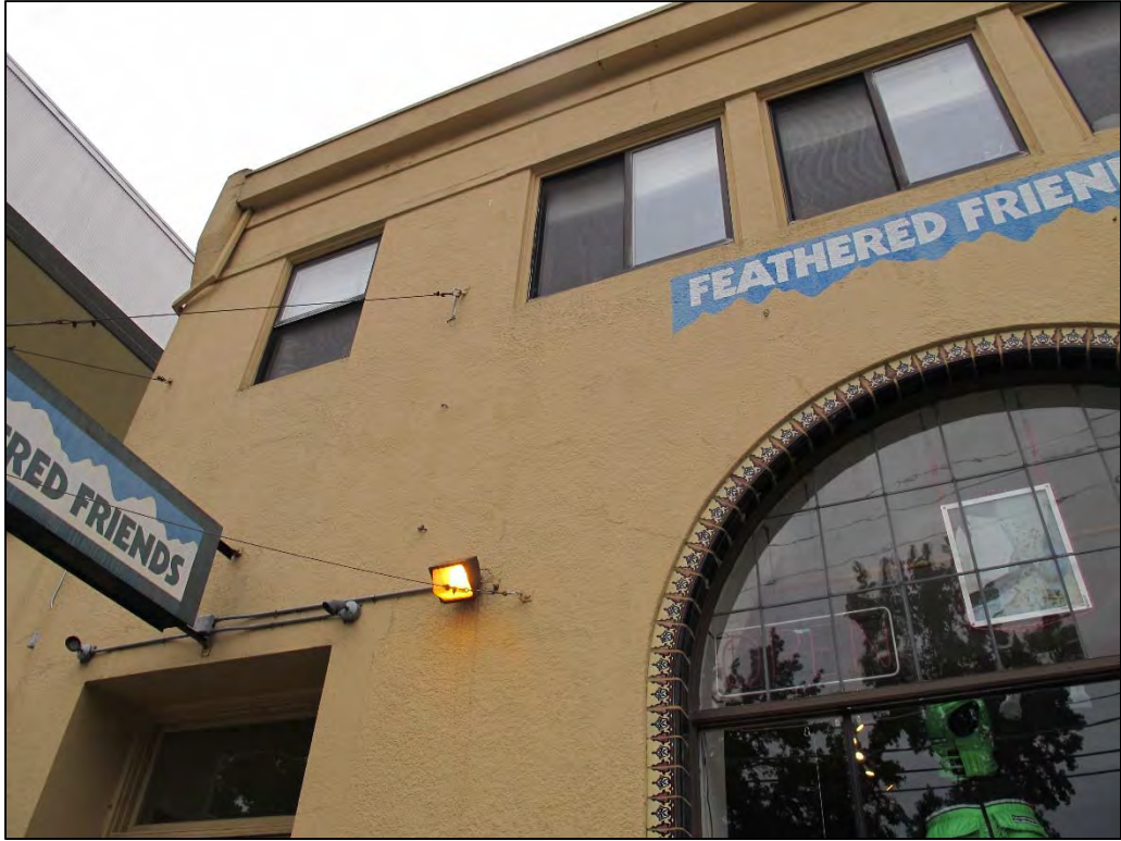
Fig. 47 – East elevation, detail
