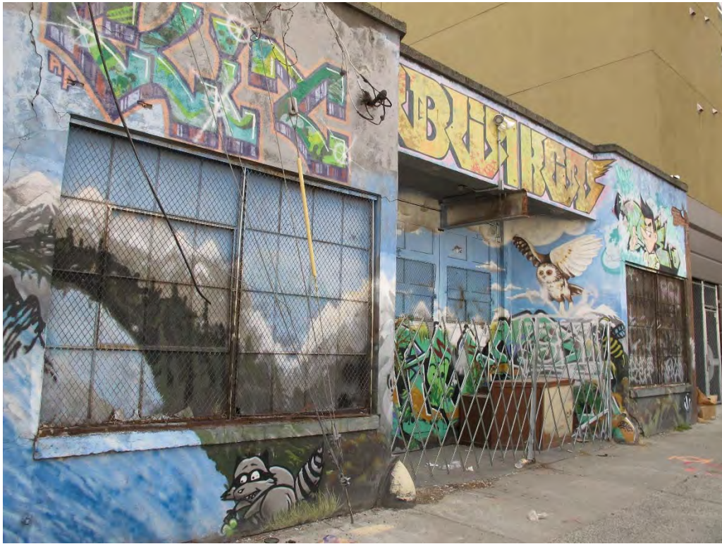
Fig. 65 – West elevation, detail. Note wide flange beam above double doors for traveling hoist.
