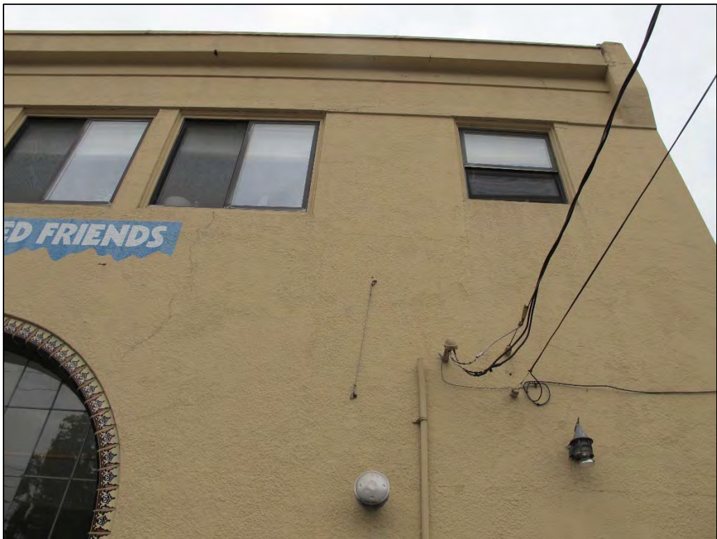
Fig. 48 – East elevation, detail
