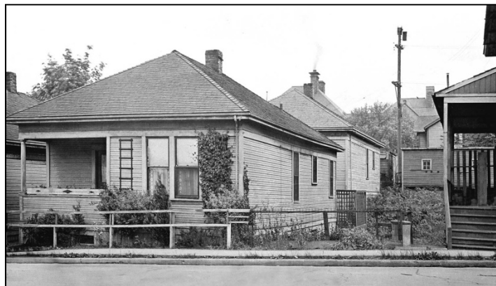
Fig. 10 – Typical Cascade worker cottages in 1937. Located at northeast corner of Minor Avenue and Thomas Street; these were part of the Fairview Homestead Association for the Benefit of Mechanics and Laborers Addition to the City of Seattle. The Cascade School visible in the distance. (Tax assessor photo, via www.pauldorpat.com )
