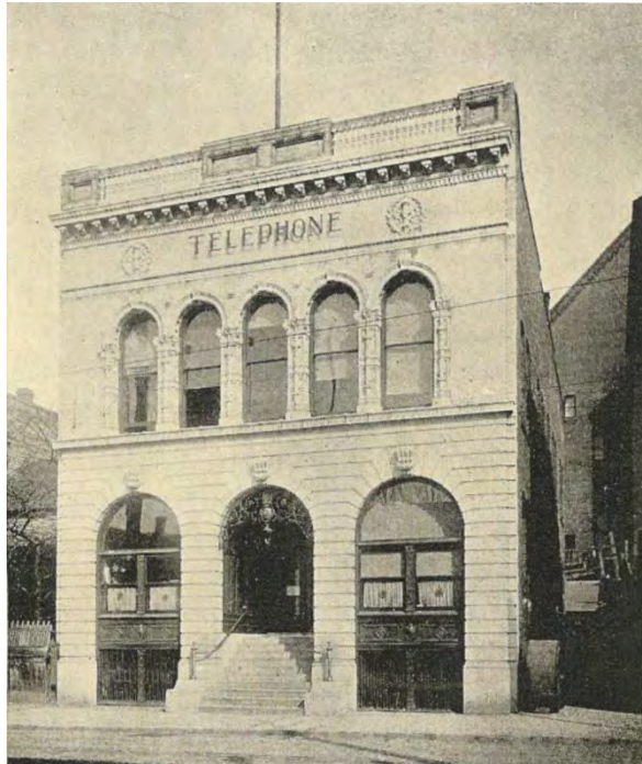
Fig. 16 – Sunset Telephone & Telegraph Company exchange building at 1108 3 rd Avenue (b. 1900). Sunset later became Pacific Telephone and Telegraph Company in 1917.
