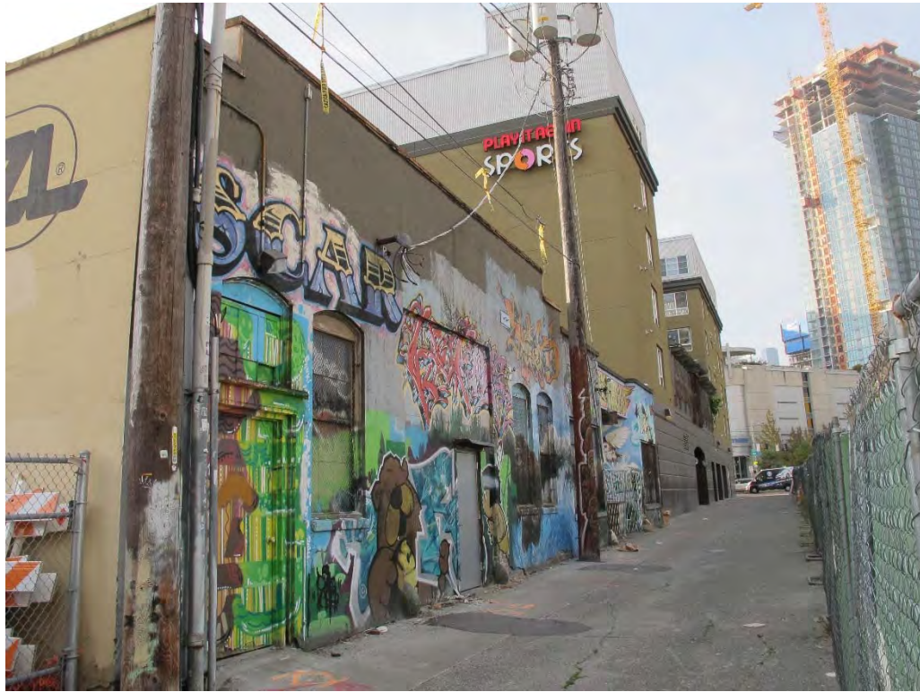
Fig. 61 – West elevation, north part
