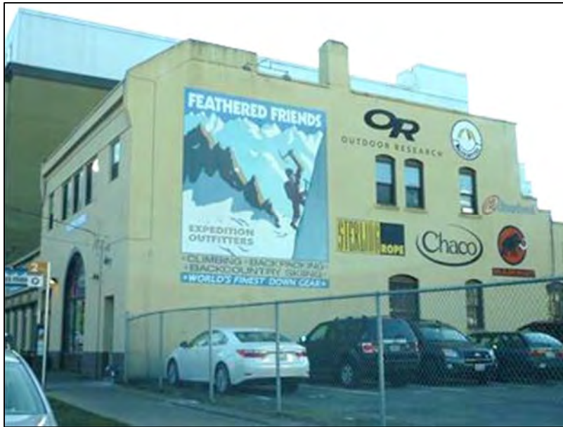
Fig. 39 – Tax assessor photo, c. 2008, showing unobstructed view of east part of north elevation. (King County Tax Assessor; original image poor)
