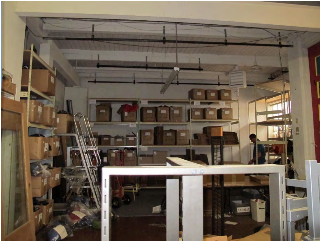
Fig. 94 – Interior, storage space in southwest building corner.
