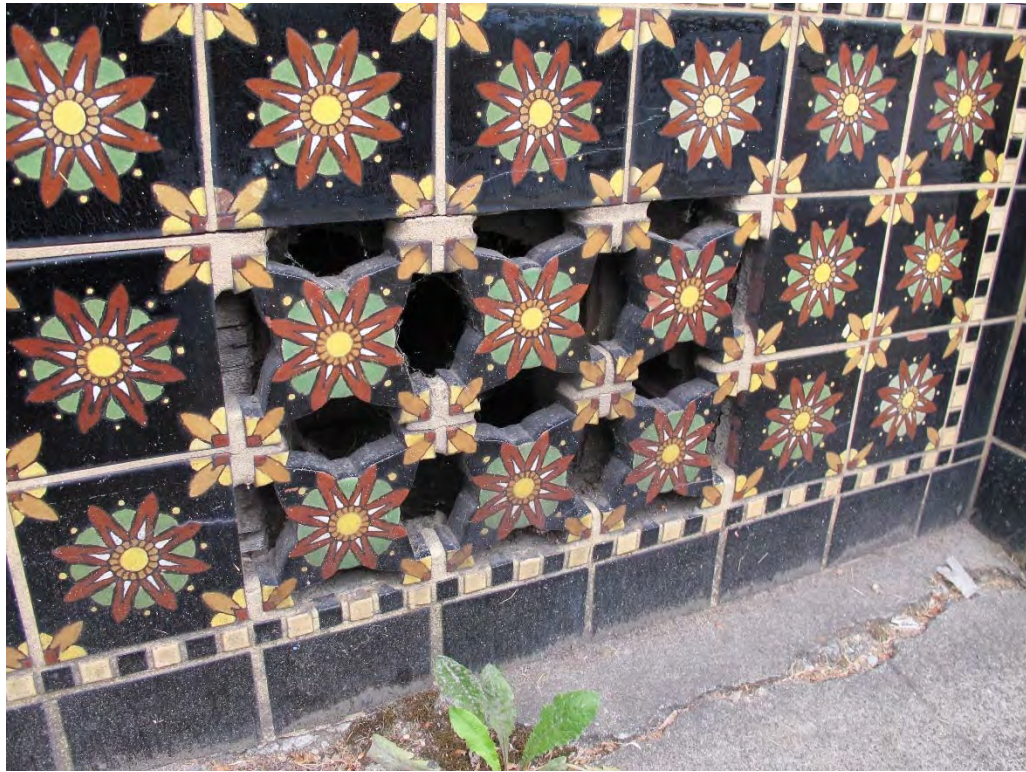
Fig. 49 – East elevation, detail of tile, arched window bulkhead. Tiles cut for vent.
