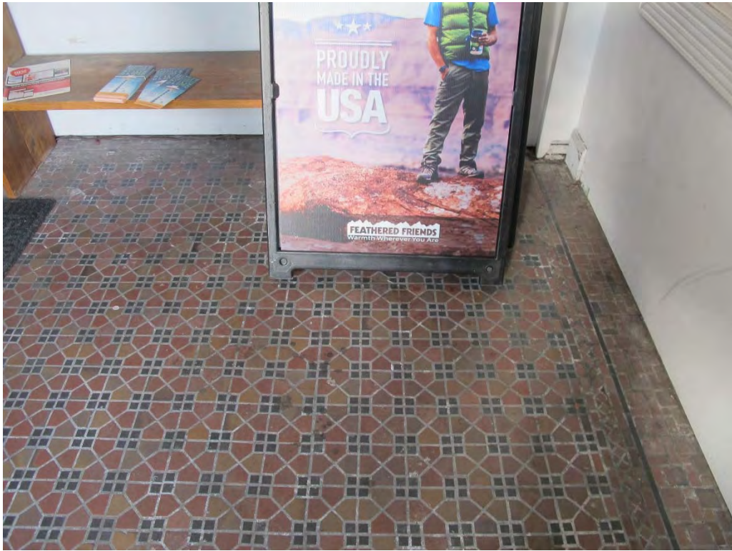
Fig. 69 – Tile at main entry vestibule
