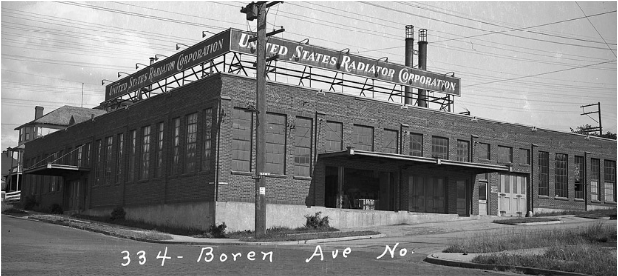
Fig. 31 – United States Radiator Corporation building (1925), at 334 Boren Avenue North; a designated Seattle landmark. (King County Tax Assessor)
