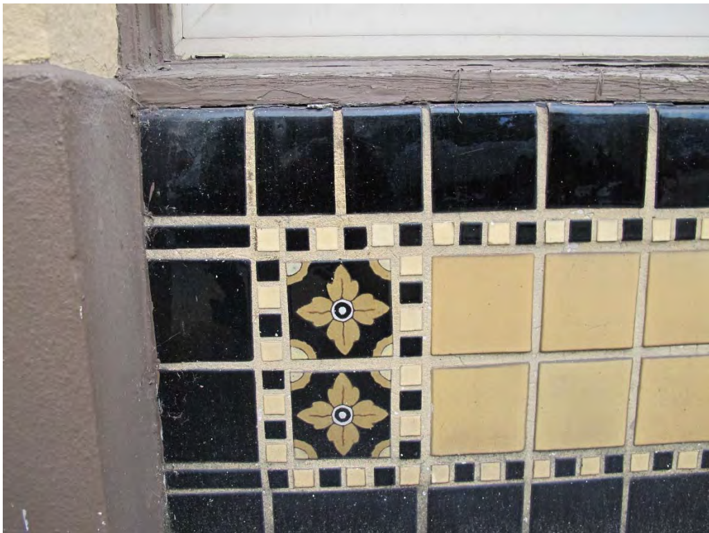
Fig. 54 – East elevation, detail of tile.
