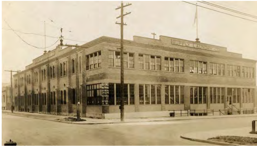
Fig. 8 – Supply Laundry in 1917, typical of several laundries in the neighborhood. Located at the southwest corner of Yale & Republican. (MOHAI Webster & Stevens Collection 2010-52-2)
