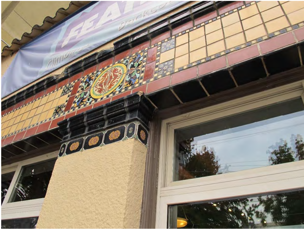
Fig. 53 – East elevation, detail of tile.
