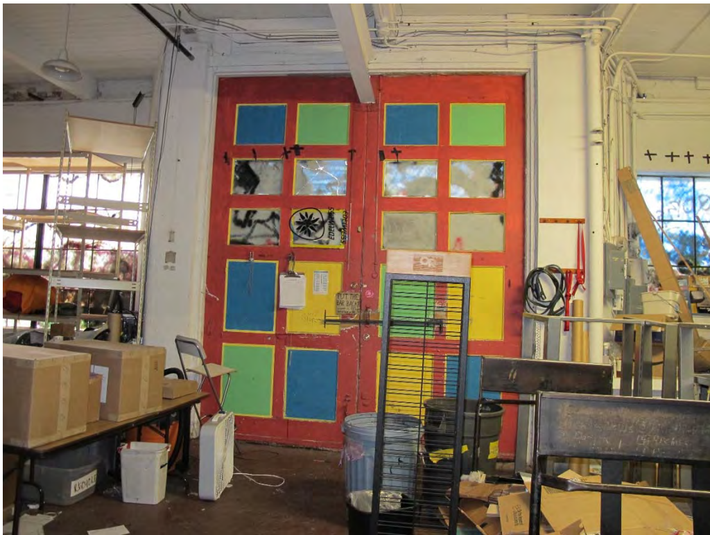
Fig. 92 – Interior, storage space in southwest building corner. Note wide flange beam above double doors for traveling hoist mechanism.
