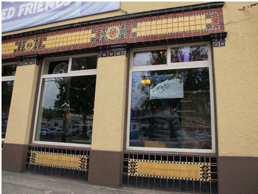
Fig. 52 – East elevation, detail of tile.
